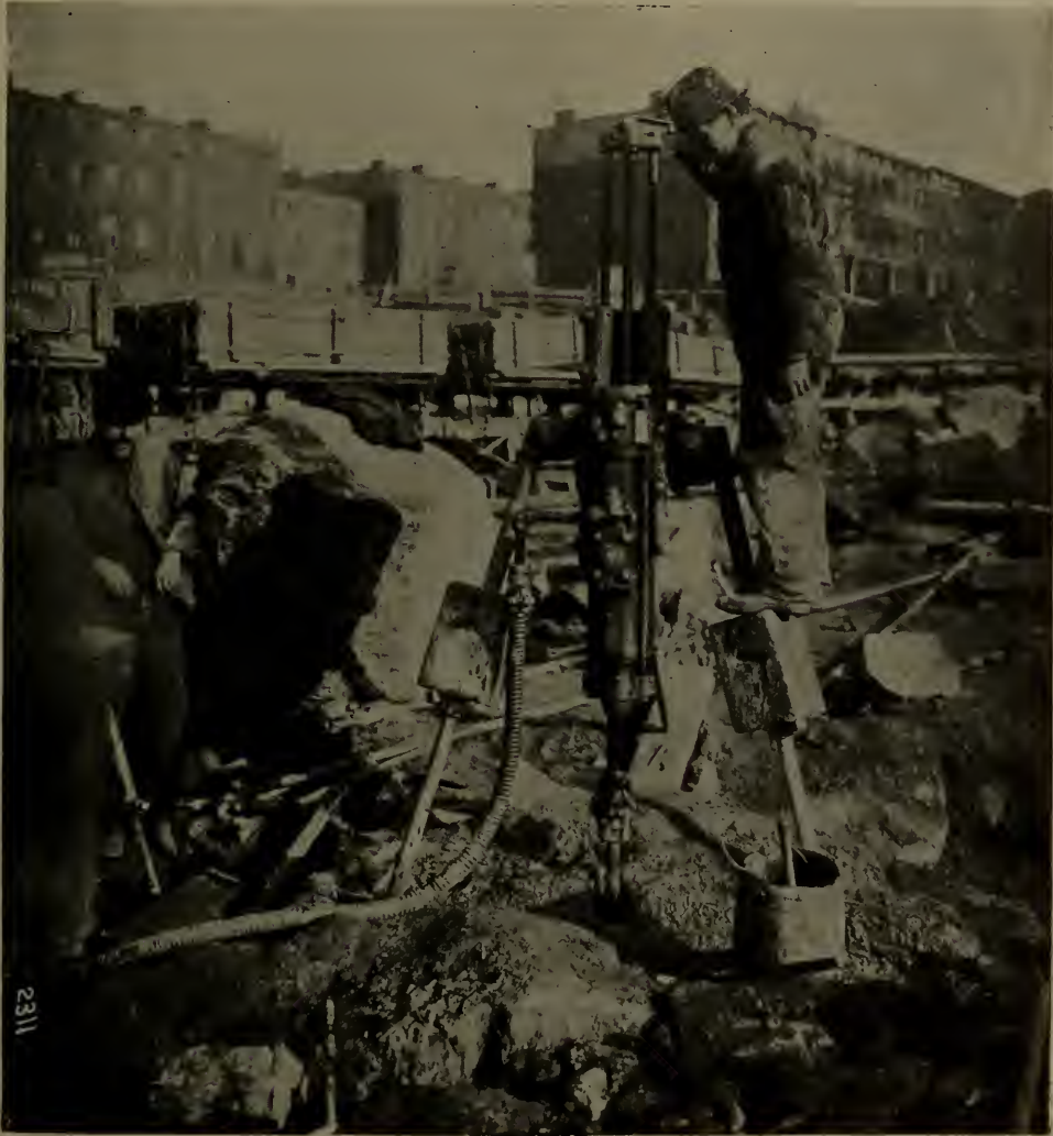
Drilling for P. R. R. Terminal Excavation.
